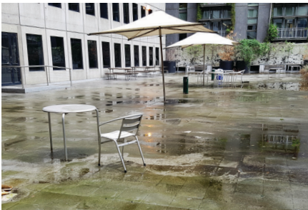
Existing liquid membrane applied over tiles prior to works commencing.
